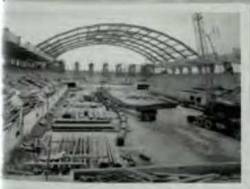
Coliseum Under Construction (c.1959)
