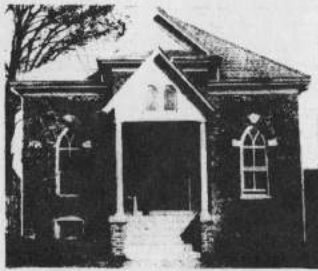
CITY'S FIRST SYNAGOGUE WAS ON EAST LEE STREET
